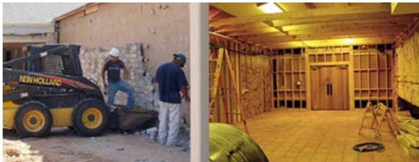
Crews began demolishing the old Texas Ranger Research Center last month. In the photographs above, workers remove the exterior stone and interior wood paneling in preparation for the expansion. The original modest 900 square foot facility will expand into a modern facility of approximately 4,000 square feet with greatly expanded archives, exhibits and reading space.
