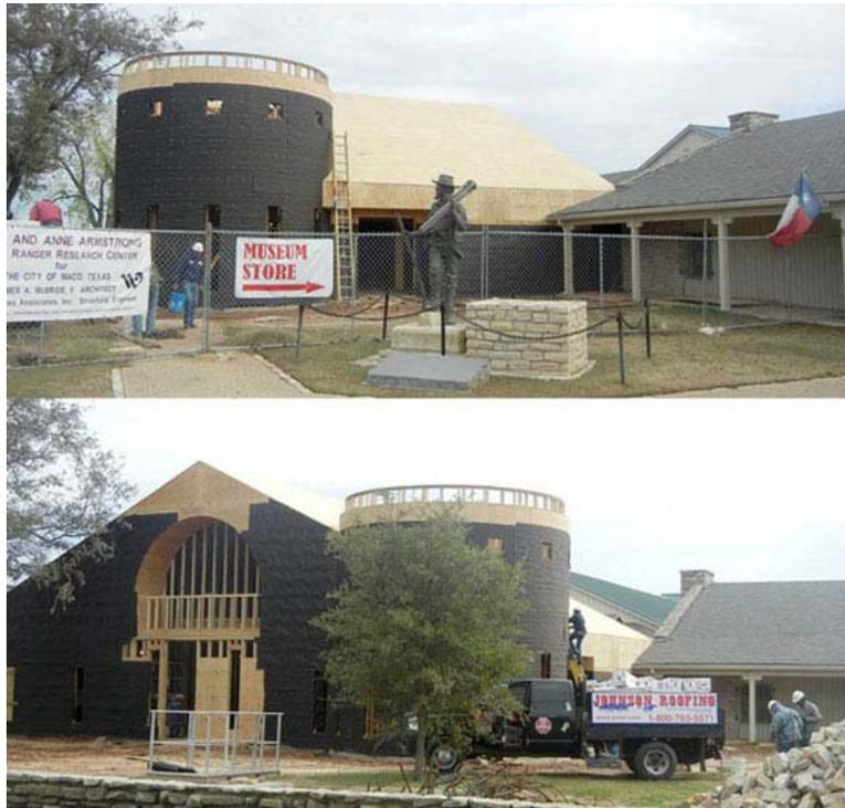
In the photographs above, workers nail wood sheets on top of the rafters as part of the framing of the Research Center roof.
